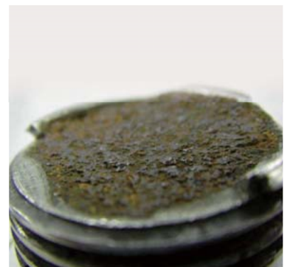
③ Breakage of bolt
